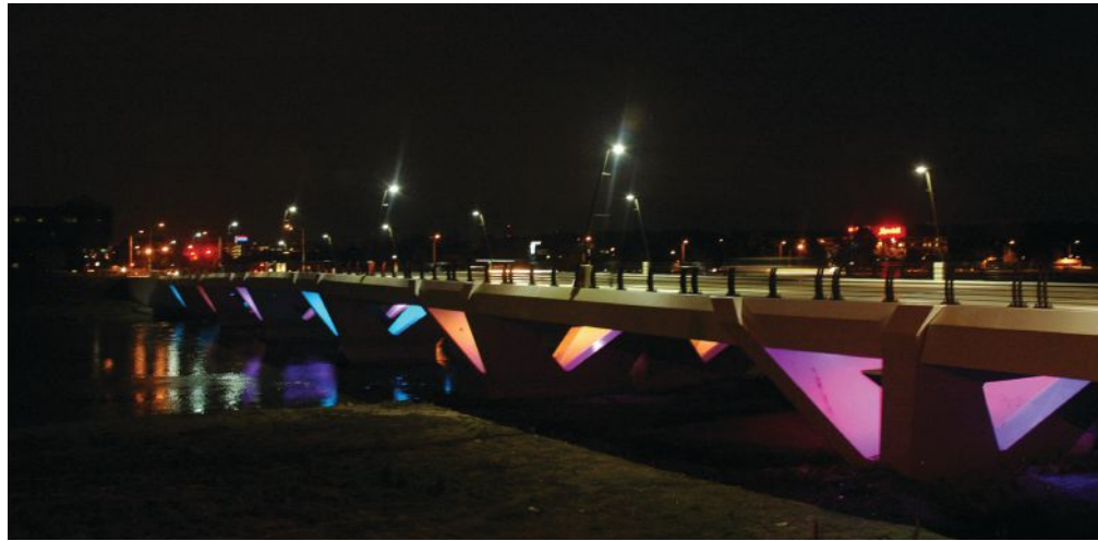
Figure 3. Colored LED lighting within the V-shaped piers of the Stewart Street Bridge enliven the nighttime appearance of the Great Miami River in Dayton, Ohio. Photo: Woolpert Inc.
