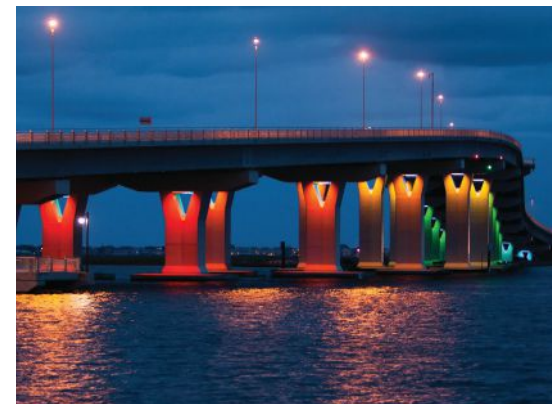
Figure 5. Timed sequences of color change in the LED pier lighting produce the illusion of waves of color moving across Great Egg Harbor Bay. Photo: Michael Baker International.
