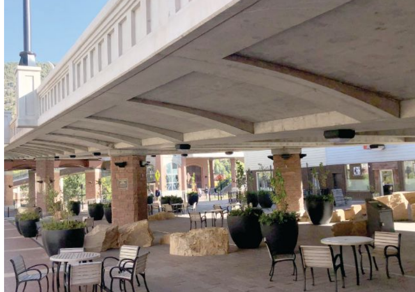
Shading on the tapered overhangs produces a visually thin superstructure. The stone finish on the columns matches the color of the mountains in the area.
