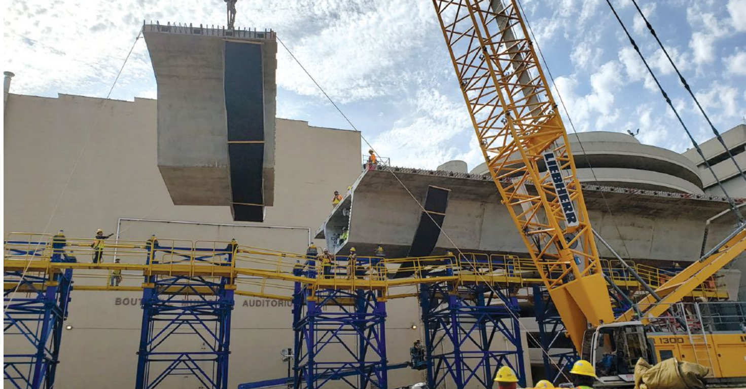
Erection of a precast concrete box-girder segment on temporary support towers for the first span of the central business district bridges. Photo: Volkert Inc.
