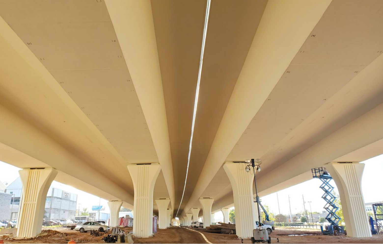
The area beneath the completed mainline spans after painting. City officials intend to use this area for public events. Photo: Johnson Bros.
