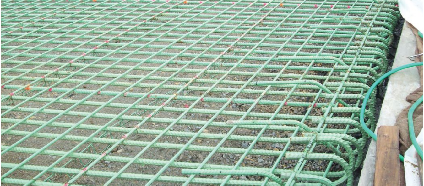
With proper inspection and handling, epoxy-coated reinforcing steel effectively protects against corrosion in reinforced concrete applications such as this bottom mat of reinforcement for a bridge approach slab.
