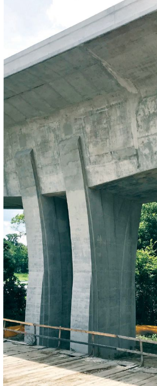
A dual-shaft pier was used to stabilize the pier segment. Photo: Superior Construction Company Southeast.
