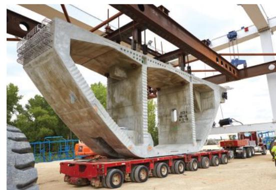
The precast concrete bridge segments for the St. Croix bridge were cast in two locations: The smaller segments were made on site and were handled with a self-propelled modular transporter. The larger segments were cast and stored on Grey Cloud Island, downstream from the project. Segments were surveyed three times in the casting yard by two different parties to ensure accuracy of casting.
