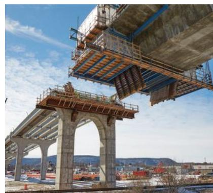
To facilitate the project schedule, the Minnesota Department of Transportation chose Ames Construction as construction manager/general contractor to construct the Highway 43 Mississippi River Crossing in Winona, Minn. The approaches are prestressed concrete girder units, and the four-span main unit is a cast-in-place, balanced-cantilever segmental bridge featuring a concrete box-girder design.
