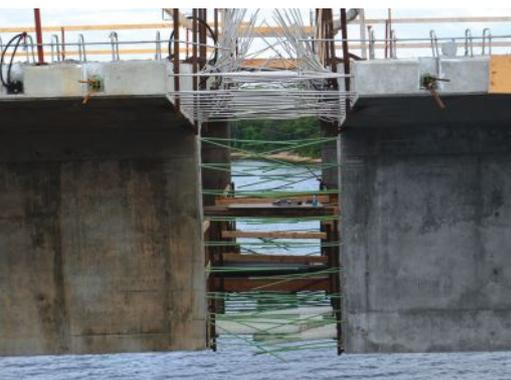
A cast-in-place closure pour for the Dresbach bridge. Stainless steel reinforcement was used in the deck, and epoxy-coated reinforcement was used in the box-girder webs and bottom slab. Post-tensioning ducts at the bottom of the web and anchorages for multistrand slab tendons are also visible.
