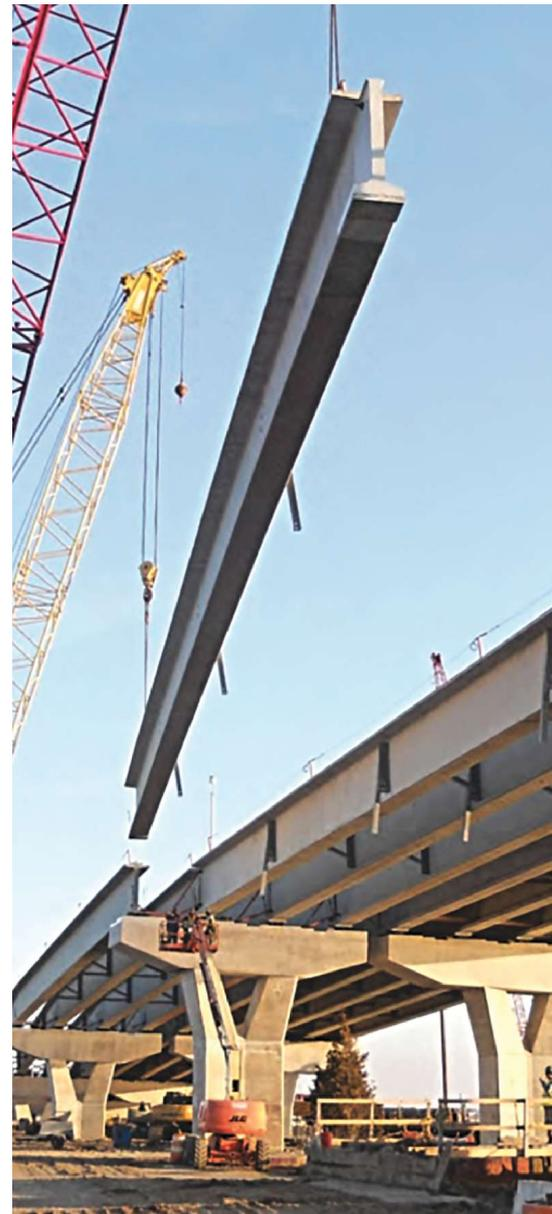
altering stresses and reducing initial camber and camber growth. The beneficial effects of moving the lifting points away from the girder ends are also discussed.
