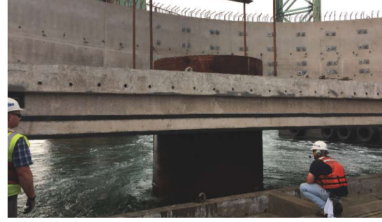
Nose unit installation over a drilled shaft. Photo: Cianbro.
