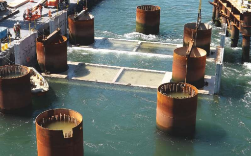
Installation of the drilled-shaft units. Photo: Cianbro.
