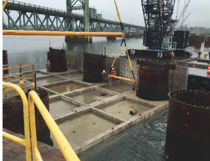
Fill unit installation. Photo: Cianbro.
