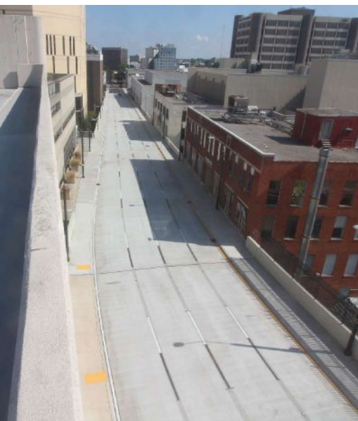
The completed Courtland Street Bridge.
