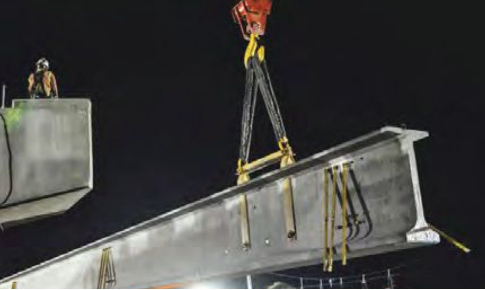
Figure 3. Example of extended rigid lifting system. Photo: The Lane Construction Corporation.
