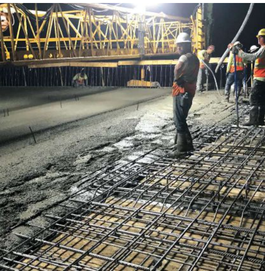
Nighttime placement of lightweight concrete with polyfibers for the bridge deck. Photo: Ric Maggenti.
