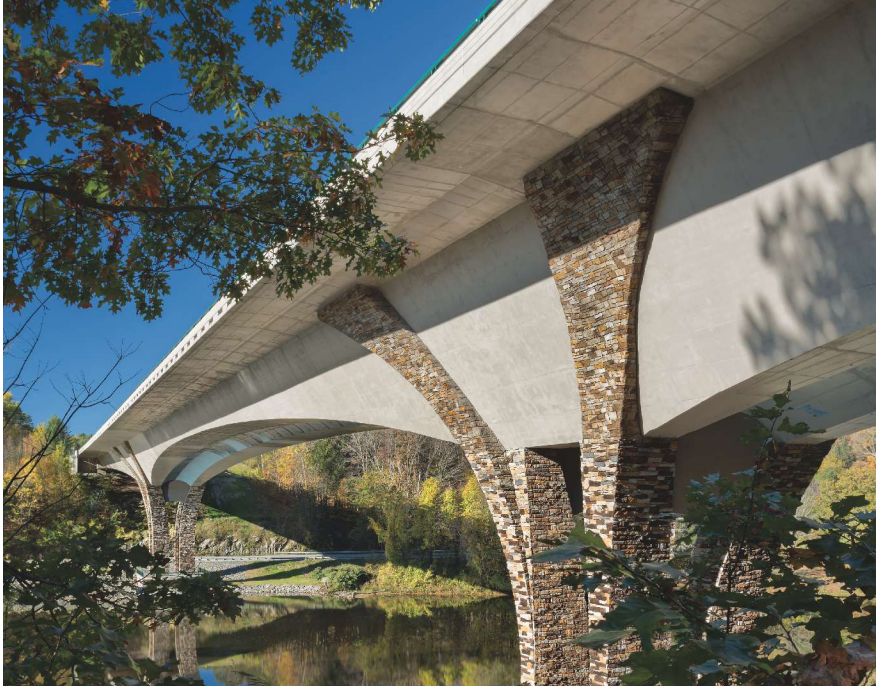
The new gateway bridge in Brattleboro, Vt., carries Interstate 91 over the West River, Vermont Route 30, and the West River Trail. Located in southern Vermont, the bridge provides a visual “gateway” to the state’s mountains, valleys, and rivers.
