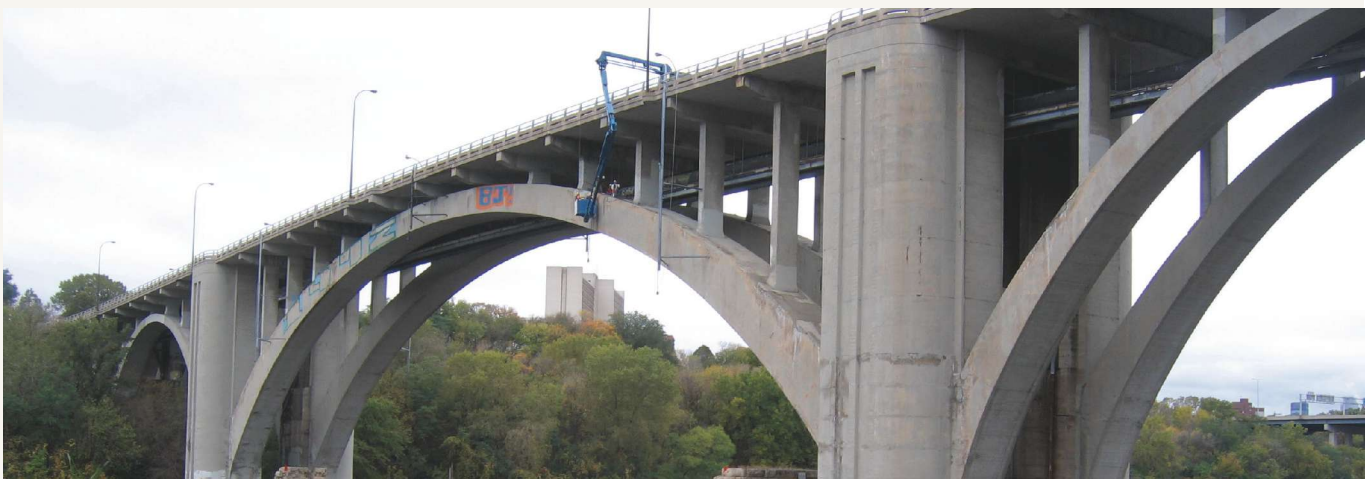
Franklin Avenue Bridge during condition investigation by snoopers truck. Photo: WJE.
