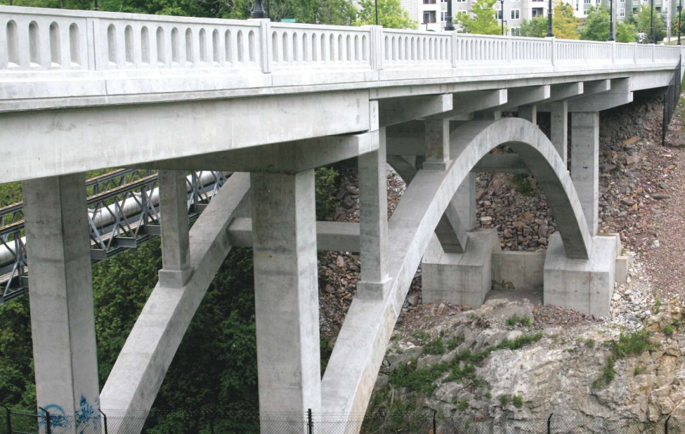
In an effort to replicate the aesthetics of the original Lime Kiln Bridge over the Winooski River Gorge, which was one of the first open-spandrel arch bridges in the United States, designers used precast concrete beams along with cast-in-place concrete arches, piers, floor beams, and deck. Special attention was paid to the visual depth of the arch spans, the depth of intermediate spans, and the post spacing on railings. Photo: VHB-Vanasse Hangen Brustin.
