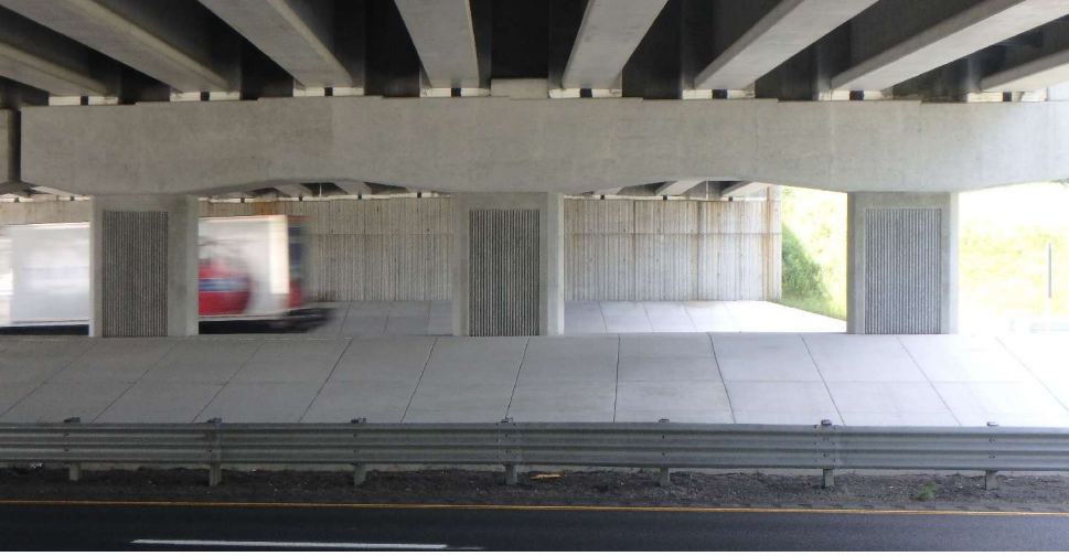
View beneath completed bridge showing the center pier and abutment.
