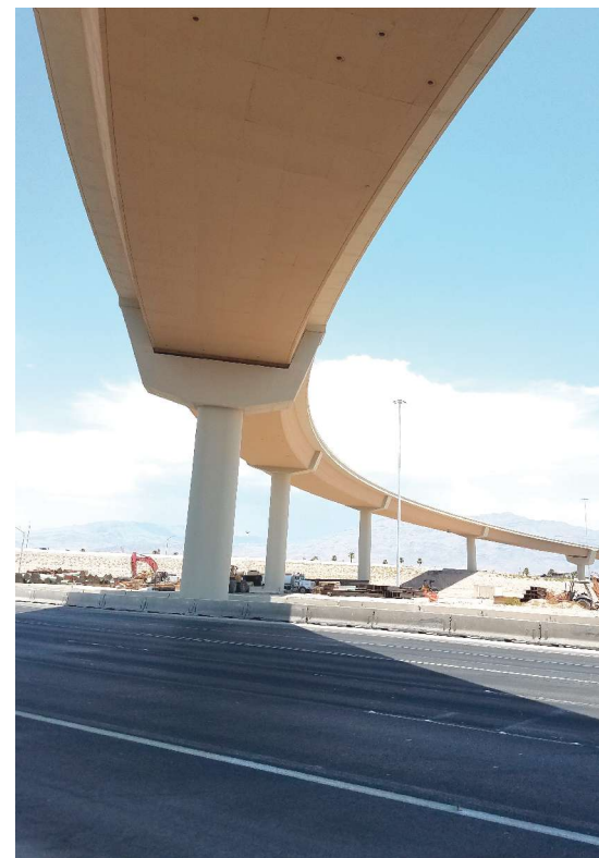
Completed Westbound Clark County Route 215 to Southbound U.S. Route 95 Flyover Bridge. Photo: Nevada Department of Transportation.
