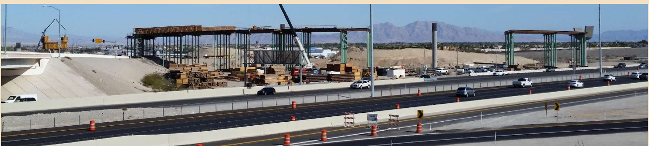
Progress photo of placement of falsework for frame 2. Photo: Nevada Department of Transportation.
