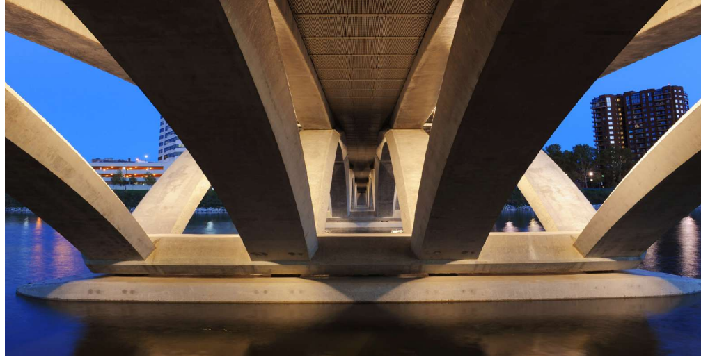
The five-span Rich Street Bridge in Columbus, Ohio, is supported on four lines of post-tensioned precast concrete arches. Photo: Randall Scheiber.
