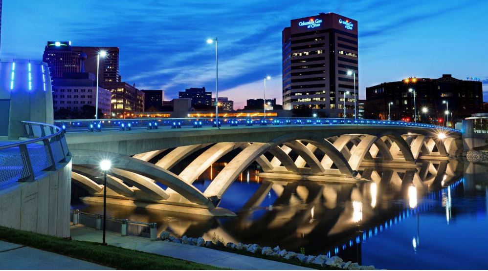
The lighting design of the Rich Street Bridge over the Scioto River in Columbus, Ohio, was developed by Gottemoeller. Photo: Randall Scheiber.
