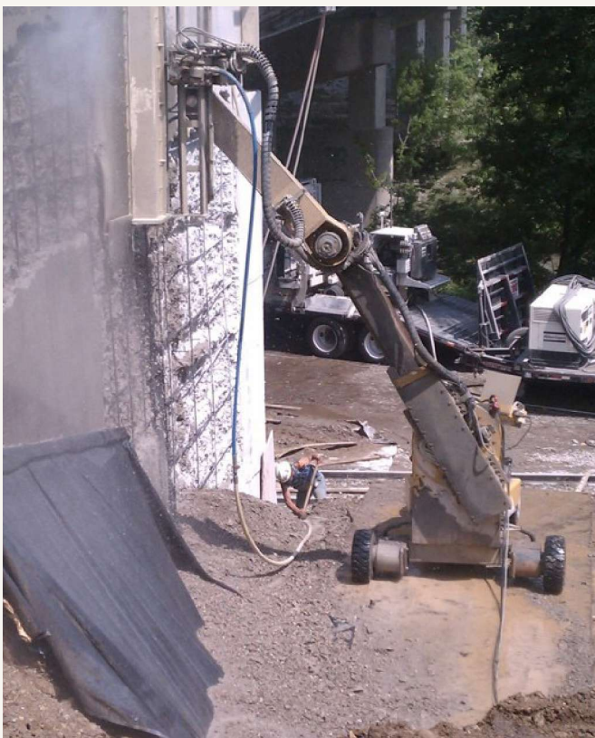
Vertical hydrodemolition of a turnback bridge abutment.
