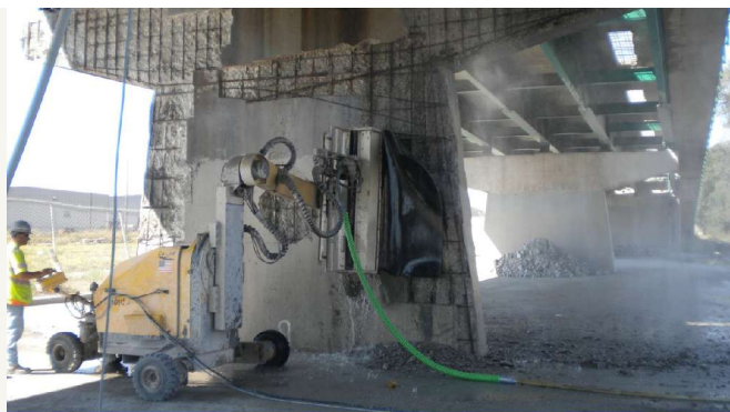
Vertical hydrodemolition of a bridge hammer-head pier.
