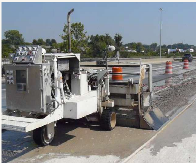
Hydrodemolition robot working on a bridge deck. All Photos: Edward Liberati.
