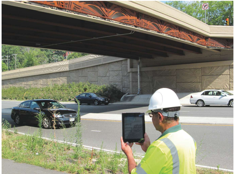
A bridge inspector uses the Bridge Inspector's Reference Manual Application on his tablet. All Photos: Federal Highway Administration.
