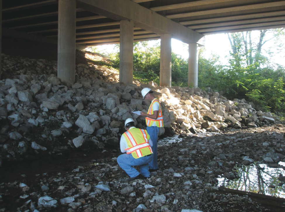
A bridge being subjected to a safety inspection.
