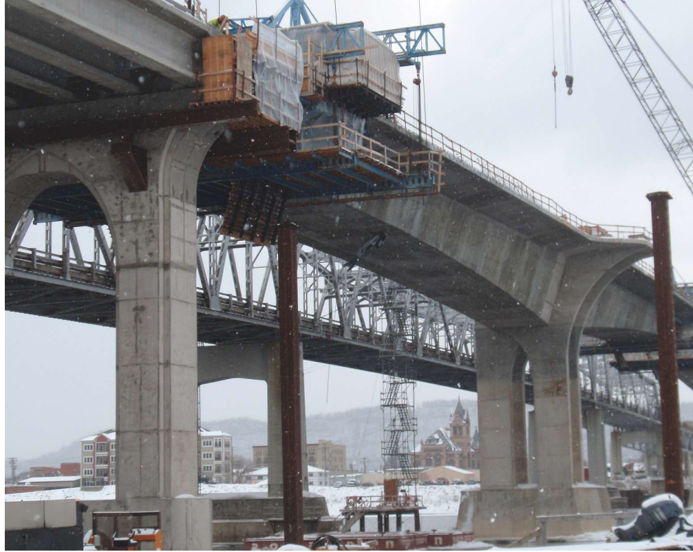
Form travelers with suspended heated enclosures enabled concrete for the segments to be placed throughout the winter. Photo: FIGG.
