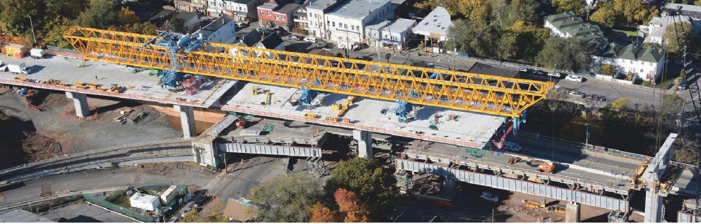
Balanced-cantilever construction for the Bayonne Bridge approaches.
