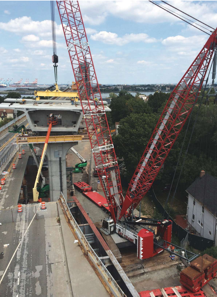
Tight constraints for erection of single-cell box-girder pier table segment. The 42-ft difference in the elevations of the old and new approaches is evident. All Photos and Figures: HDR.
