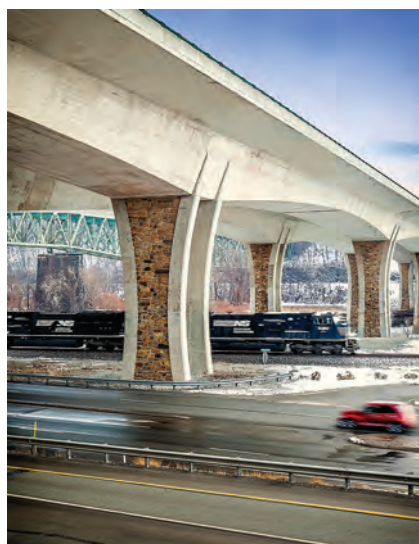
Walsh Group built the Allegheny River Bridge, which features twin cast-in-place concrete segmental bridges with 532-ft-long main spans. Photo: FIGG.
