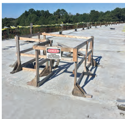
Signs help identify confined spaces to workers or inspectors not directly involved with an operation. Photo: Andrew Mahoney.
