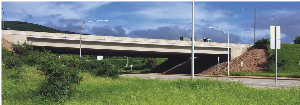
The North-South Road on Oahu features twin 165-ft-long, single-span, integral-abutment bridges with post-tensioned, spliced girders and precast concrete deck panels.
