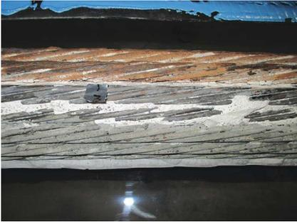
Corroded strands in a bonded post-tensioning tendon.
