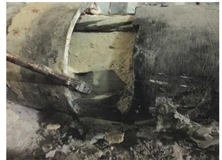
Segregation of grout (light tan is soft and grey is solid) and void at top of tendon.
