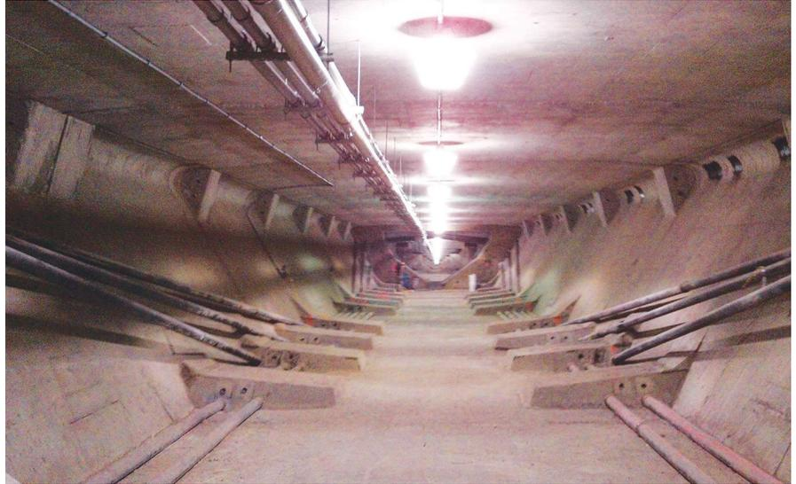
Example of a post-tensioned, box-girder bridge with external post-tensioning tendons. All Photos: Vector Corrosion Technologies Ltd.
