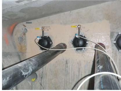
Impregnation of post-tensioning tendon from end anchorage.
