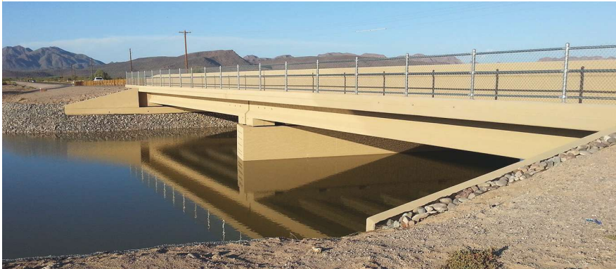
Completed Gila River Bridge. Photo: Greg Harasha.
