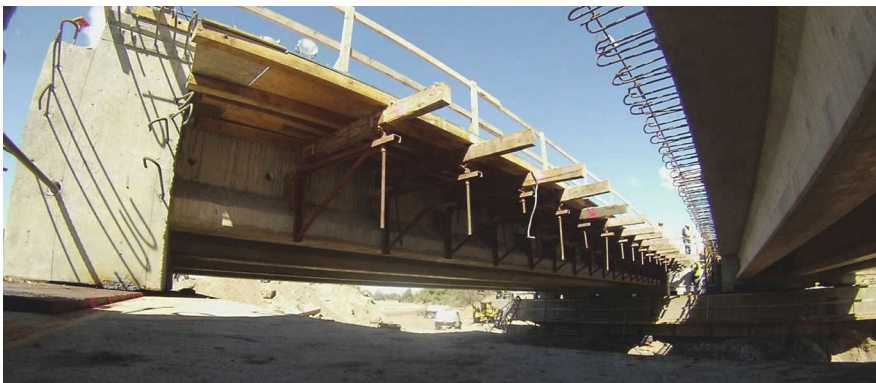
Last segment of bridge sliding into place. Photo: Shawn Sheble.
