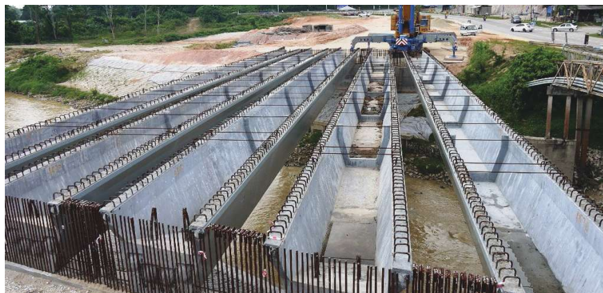
Figure 2. Rantau-Siliau Bridge during construction.
