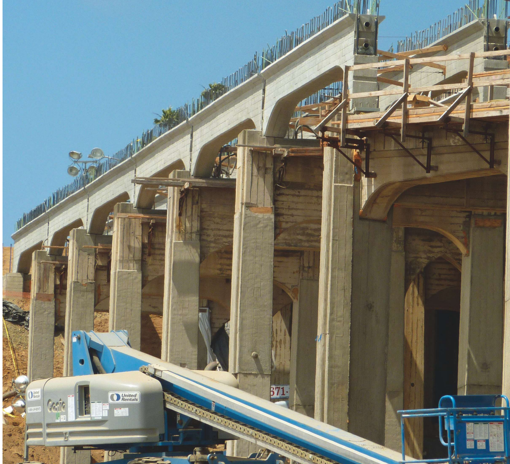
Precast concrete girders erected on rehabilitated substructure.
