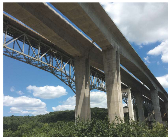
The 2252-ft-long, twin six-span structures of the Jeremiah Morrow Bridge in Warren County, Ohio, feature post-tensioned, single-cell box girders. The existing steel truss bridge will be removed now that the two concrete spans are complete. Photo: OmniPro Services.
