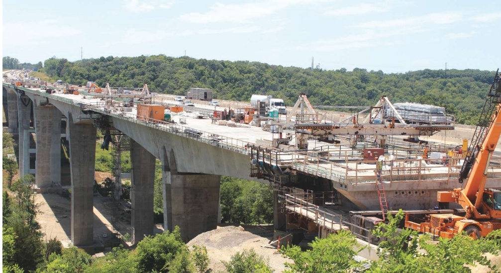
The Jeremiah Morrow Bridge is the tallest bridge in Ohio at 239 ft above the valley floor, and the first cast-in-place, concrete segmental box-girder structure owned by the Ohio Department of Transportation. Photo: OmniPro Services.
