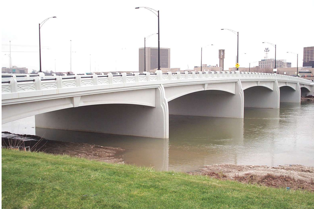
The 5th Street bridge-replacement project in Montgomery County, Ohio, featured self-consolidating concrete for the decorative concrete parapets to create details that offered a high-quality finish. Approximately 6250 yd 3 of structural concrete were used in the 5th Street bridge-replacement project's pilings, beams, decorative pier ends, and other components. Photo: Kokosing.
