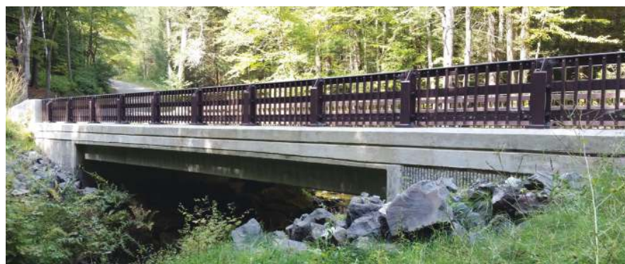
A bridge in Charlemont, Mass., was one of the first to use Northeast Extreme Tee (NEXT) precast concrete beams for an integral-abutment bridge.
