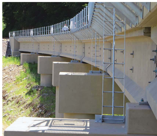
Walkway hatches provide ladder access to pier caps for inspection of beams ends and bearings. Photo: Alfred Benesch & Company.
