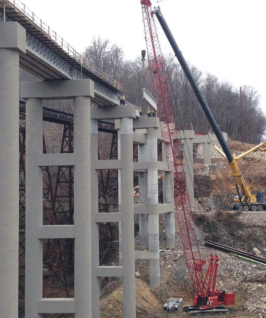
Erection of 72-in.-deep precast, prestressed concrete I-beam in an 85-ft span, using a dual crane lift. Photo: Haydon Bridge Company.
