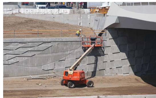
Architectural features of the Cherry Avenue Interchange including walls, abutment, and overcrossing shown during construction, prior to color staining. Photo: Tom Paiva.
