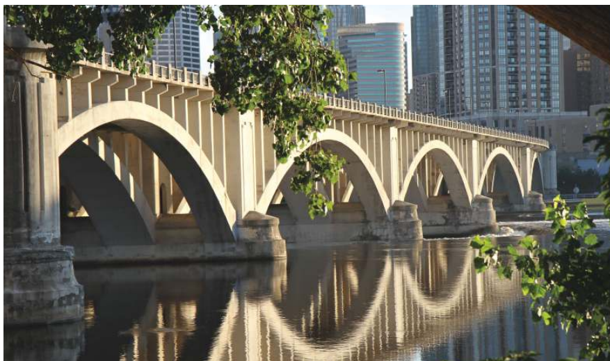
Construction on the Third Avenue Bridge in Minneapolis, Minn., began in 1914 and was completed 4 years later. It uses open-spandrel concrete arches to span the Mississippi River. Photo: John A. Weeks III.
