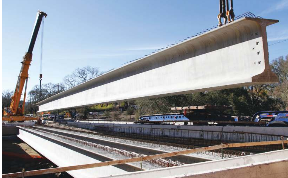
Setting last girder for stage II.
