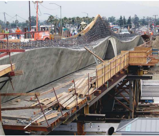
Citrus Avenue Overcrossing barrier during construction. Photo: Brett Makley.
