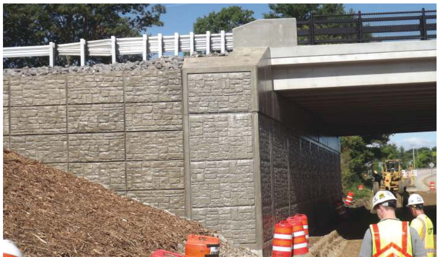
Recently completed Kittery Overpass Bridge, Kittery, Maine. This ABC project utilized precast concrete cantilevered abutments, precast concrete Northeast Extreme Tee (NEXT) Deck Beams, and precast concrete approach slabs for rapid construction. Photo: Federal Highway Administration.
