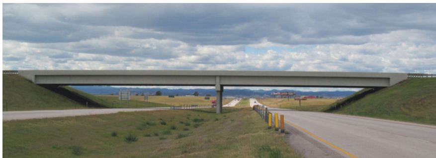
The Liberty Road Bridge over I-90, at the east entrance to Ellsworth Air Force Base, was constructed in 2002. It features eight girder lines of Type 72M prestressed concrete girders with spans of 129 and 119 ft and a 60-ft-wide roadway. Photo: South Dakota Department of Transportation.
