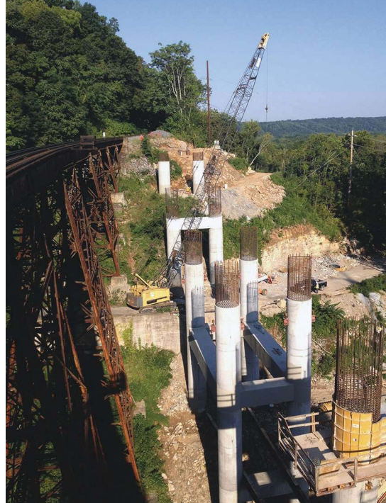
Pier construction at the west end of the bridge. Photo: P&L Railway.
