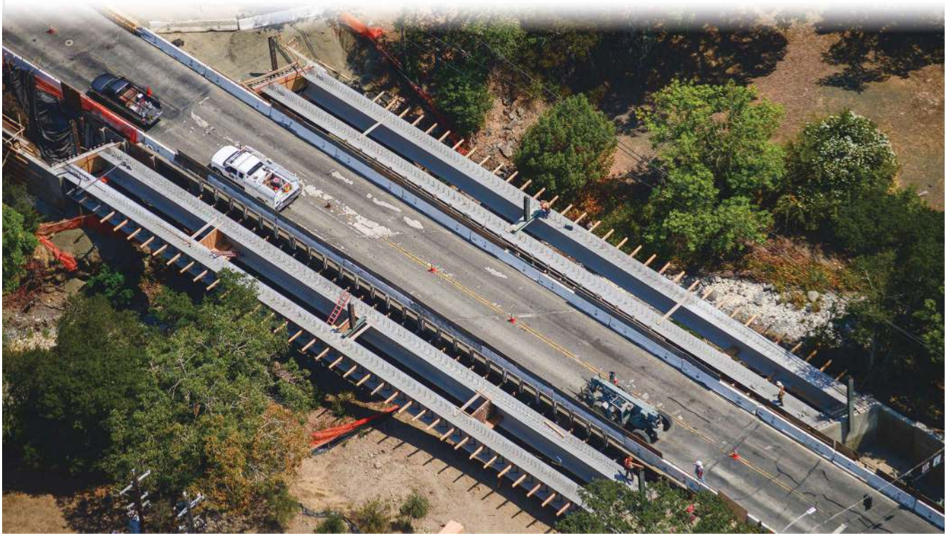
Aerial view of stage I construction, with new girders flanking the existing bridge. All Photos: Kie-Con.
