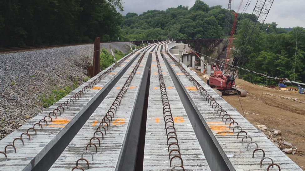
Chorded beam layout at the east end of the bridge. Photo: Alfred Benesch & Company.
