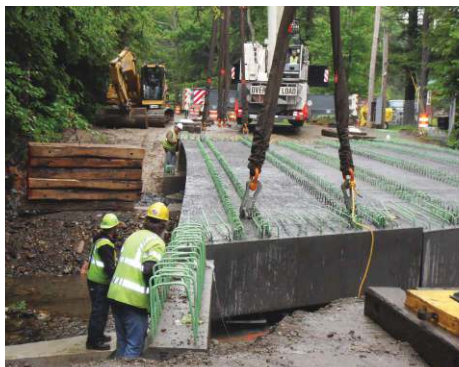
These two photographs of the Worthington Bridge in Massachusetts show the first use curved and skewed Northeast Extreme Tee (NEXT) precast concrete beams. One side of the top flange of the NEXT beam was blocked out to form the curve.
