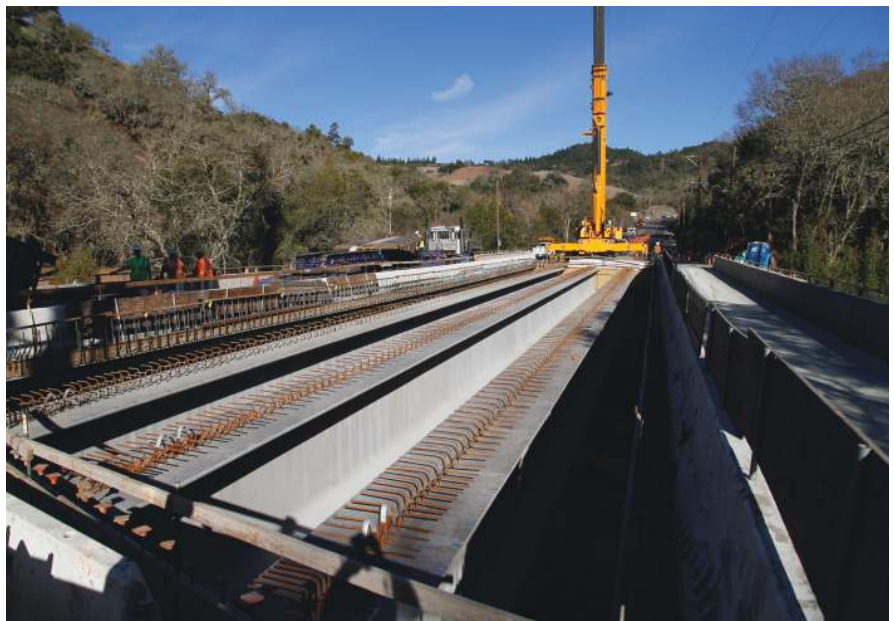
All girders set for stage II, after removal of the old bridge.
