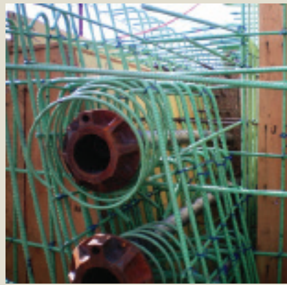
15a) Post-tensioning anchorages are installed in abutment diaphragms.
