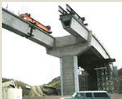
16a) Cantilevered girders are made integral with the pier. Note the drop-in girder hung from strong backs over traffic.
