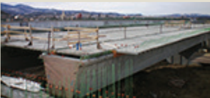
14c) Precast concrete lid slabs with deck overhang cantilevers are used with precast concrete stay-in-place deck panels between girders on the I-25 Trinidad Viaduct. Photo: PCI.
