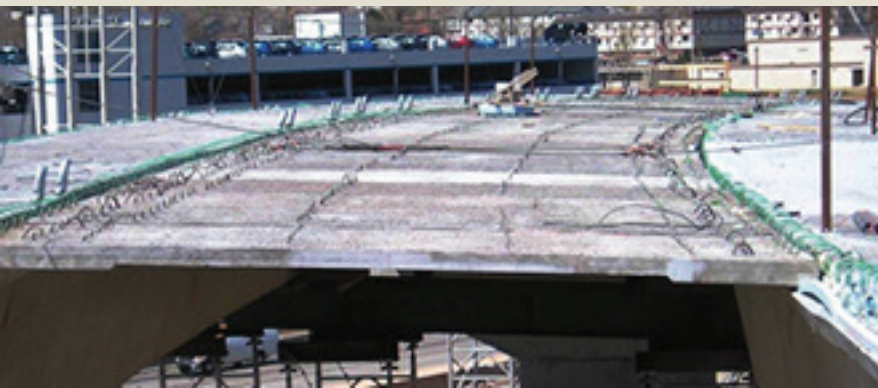
14e) Closer view of stepped-thickness precast concrete stay-in-place deck panels on a project with cast-in-place lid slabs. Photo: Summit Engineering Group.
