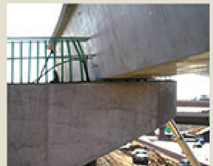
16b) The girder is supported above the pier cap where bearing grout will be inserted. Some reinforcement has been placed. Often, transverse post-tensioning extends through diaphragm and girder.
