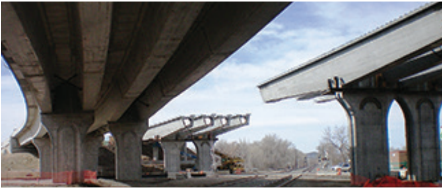
Figure 2. The I-25 Trinidad (Colorado) Viaduct features haunched girders that provide a 265-ft clear span over a rail yard. Photo: PCI.
