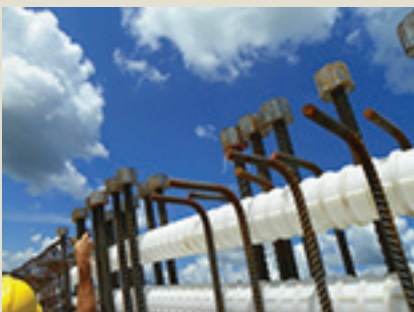
8d) No. 9 Reinforcing bars are headed at top and bottom to provide development in a short length. These bars will terminate in the cast-in-place deck.
