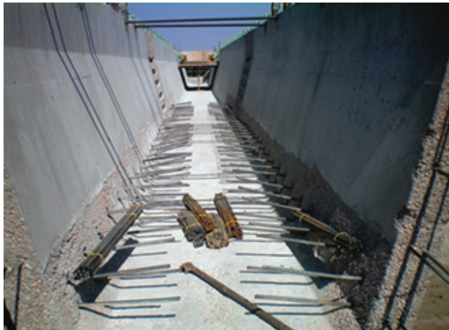
Figure 17. Threaded bars are shown inserted in form savers in the Colorado precast plant. Contact surfaces have been chemically retarded and sandblasted to improve bond with the secondary concrete cast. Photo: PCI.
