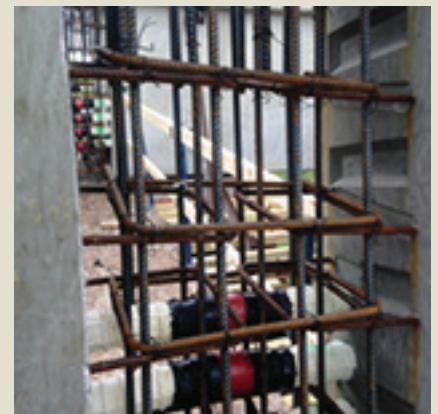
15b) Duct splices and reinforcement ready for closure placement at section splice.
