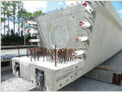
6a) The girder with tongue extension following removal from the casting form.
