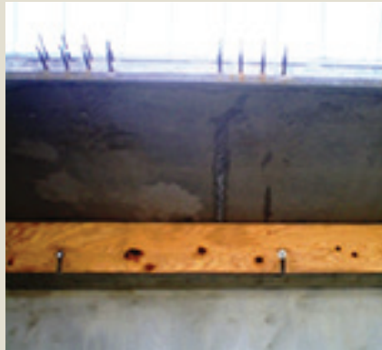
14d) Removable grout bedding form used under precast concrete deck panels like those shown in the PCI Zone 6 concept plans Photo: PCI.
