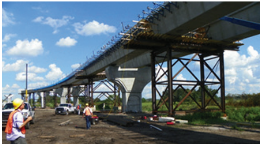
Figure 10. Engineers at TechnoQuest 2 arrive to inspect SR 417-Boggy Creek Ramp H in Orlando, Fla. Single temporary towers are located at girder splices. Towers rest on spread footing foundations. Photo: J Dick Precast Concrete Consultant.
