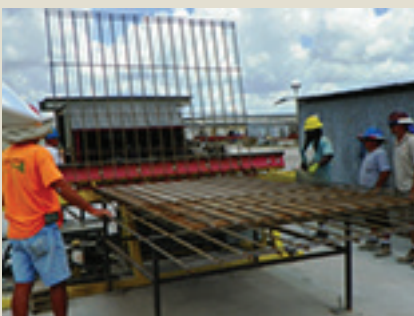
8b) Workers use a custom bending machine to fabricate special welded-wire reinforcement of No. 5 bars.
