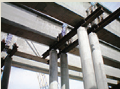
13b) The I-25 Trinidad Viaduct used temporary, cast-in-place concrete columns to support the girders at splices. Sand jacks on the columns support the steel positioning beams. The columns were later easily removed and discarded.
