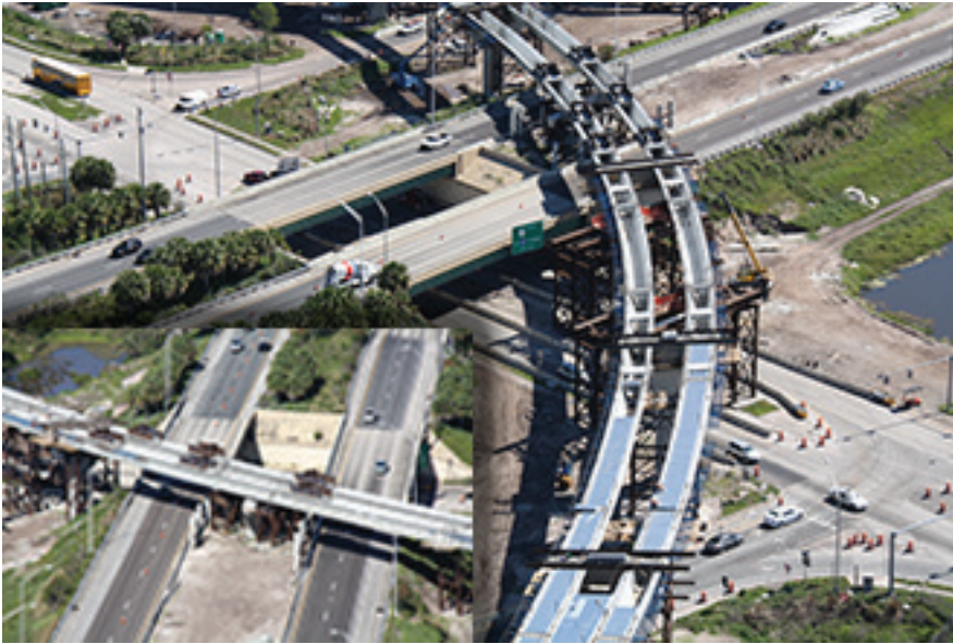
Bracing, Hold downs and strong backs at Boggy Creek Interchange. Photo: A 2 Group Inc.
