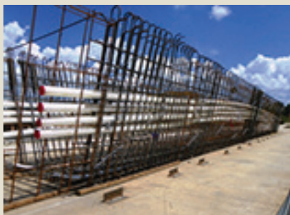
8c) Work in progress to preassemble a reinforcement cage containing post-tensioning ducts.
