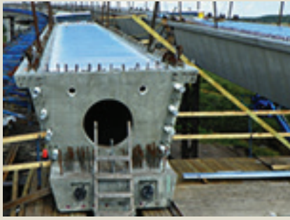
14a) Here, the CFX Project girders at the abutments are formed and ready for the cast-in-place concrete lid slabs. Photo: J Dick Precast Concrete Consultant.
