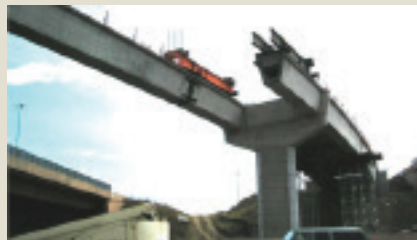
4a) Girders being erected. Note the use of strongback hangers to suspend the drop-in girders from the cantilevers over I-25.
