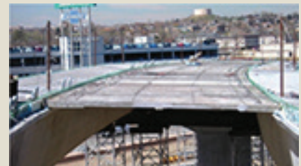
4b) Stay-in-place composite deck panels are used to span between girder flanges.
