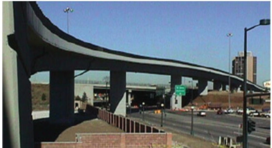
Figure 3. The Park Avenue Ramp in downtown Denver, Colo., was designed by the Colorado Department of Transportation and was precast on site. It had a maximum 230-ft-long span. The project also used 200 precast concrete stay-in-place deck panels to span between the two girder lines. Photo: Colorado Department of Transportation.
