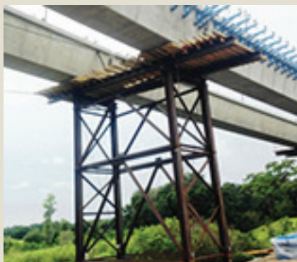
13a) Single tower used at splice location on Ramp H, CFX Project, cross-braced to withstand hurricane-force winds when only one girder is in place.
