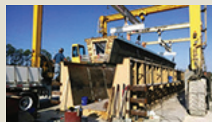
12b) A girder section being removed from its form during TechnoQuest 2. Two straddle carriers are necessary to lift the section.
