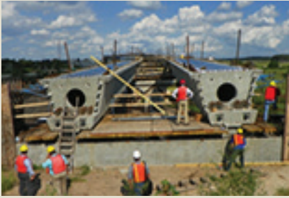
6b) Girder tongues support the girders on abutment of Ramp H, SR 416–Boggy Creek Interchange seen during TechnoQuest 2 tour.
