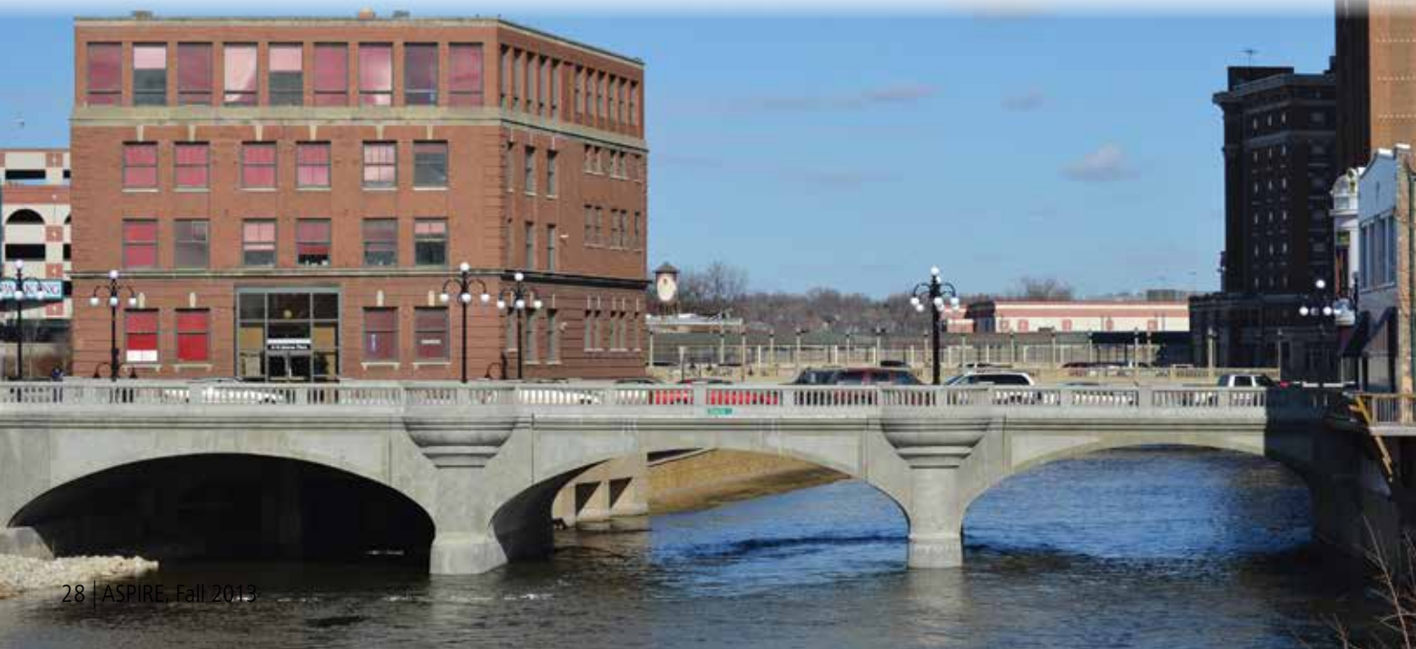
West Branch Bridge, constructed in 2012.
