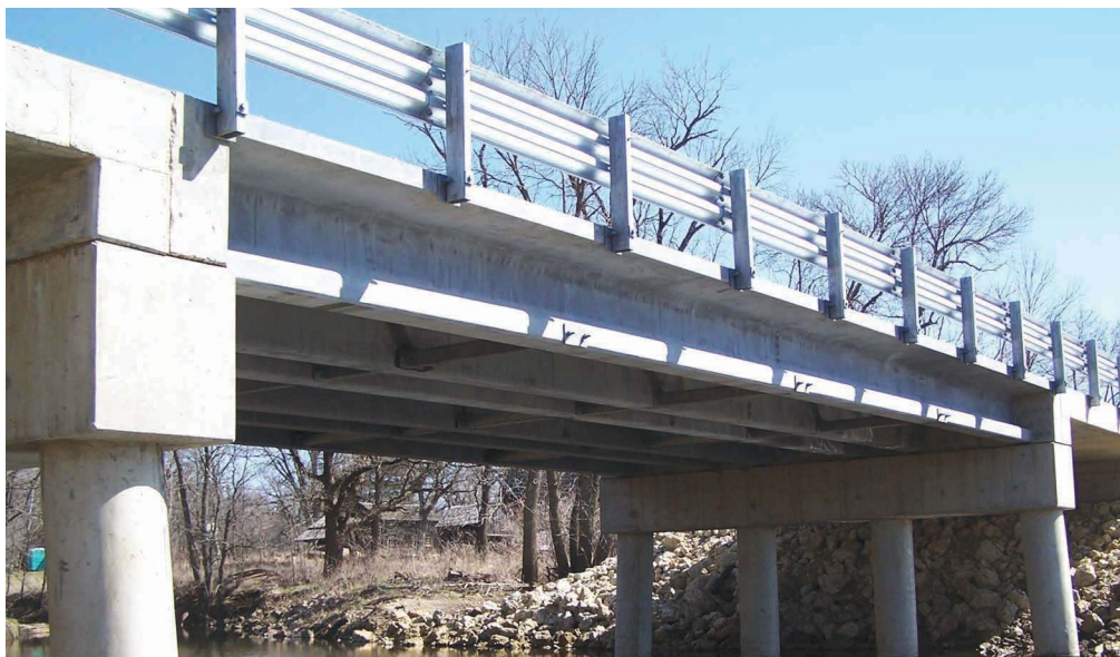
Structurally optimized, ultra-high-performance concrete, pi-girder superstructure bridge in Buchanan County, Iowa. Photo: Benjamin Graybeal, Federal Highway Administration.
