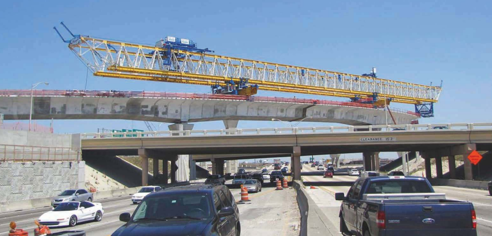
The 460-ft-long, 475-ton gantry used on the Palmetto Interchange. Photo: Condotte.
