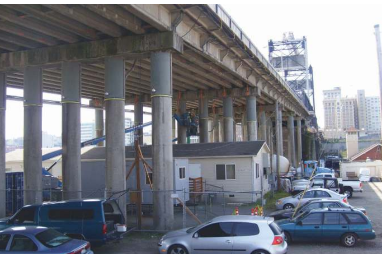
Murray Morgan Bridge port approach with repairs to the tops of the columns in place. All photos: David Evans and Associates Inc.
