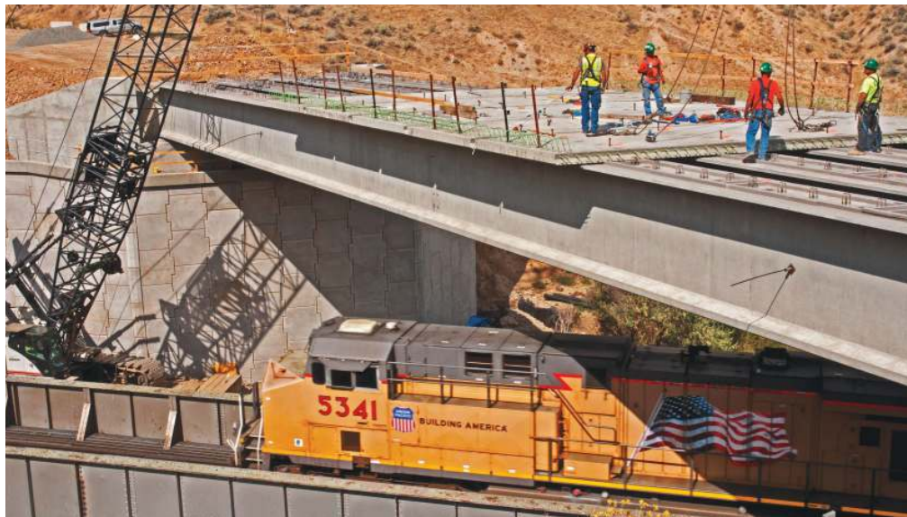
High-performance, precast concrete deck panel erection over an active Union Pacific railroad mainline. Photo: George Bornstedt.
