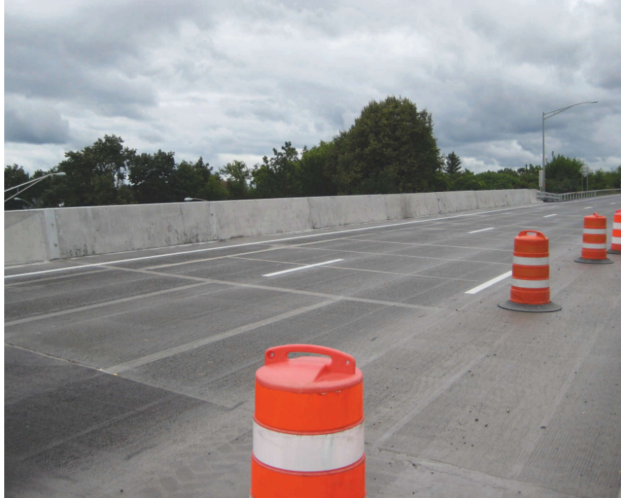
Bridge deck after grinding, grooving, and opening to traffic.
