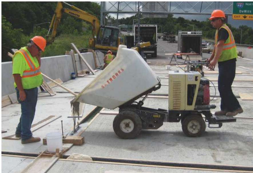
Placing operation for the field-cast, ultra-high-performance concrete. All photos: Federal Highway Administration.
