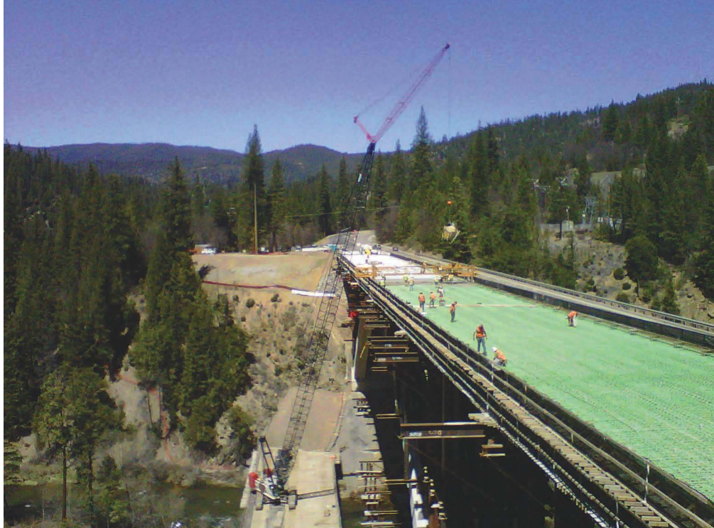
A concrete bucket on a crane was used to keep the deck placement progressing when a concrete pump truck moved to a new position.
