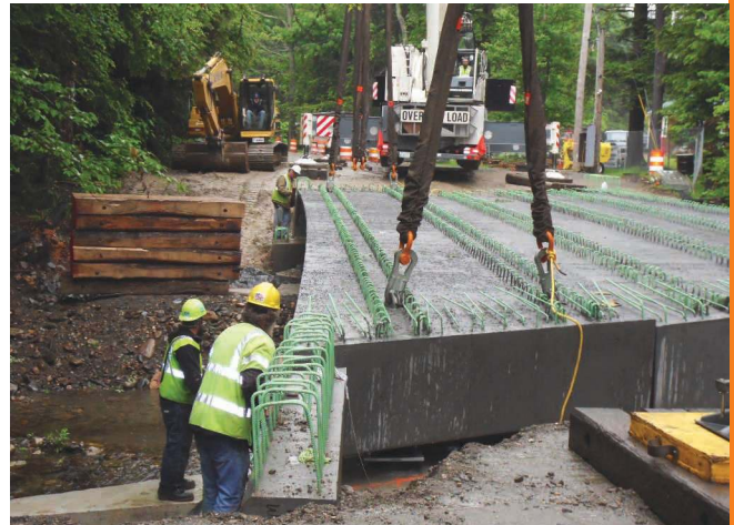
Northeast Extreme Tee (NEXT) beam installation showing the curvature of the flange. Photo: CME Associates Inc.
