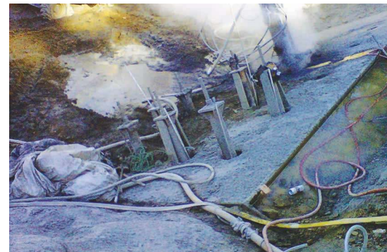
This picture shows some of the installed micropiles in the foreground and drilling in the background.
