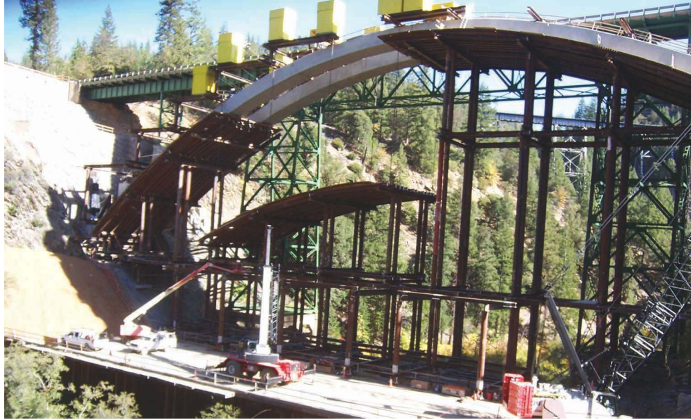
This photo shows the strand jacks mounted on the completed arches lowering the first stage arch formwork.
