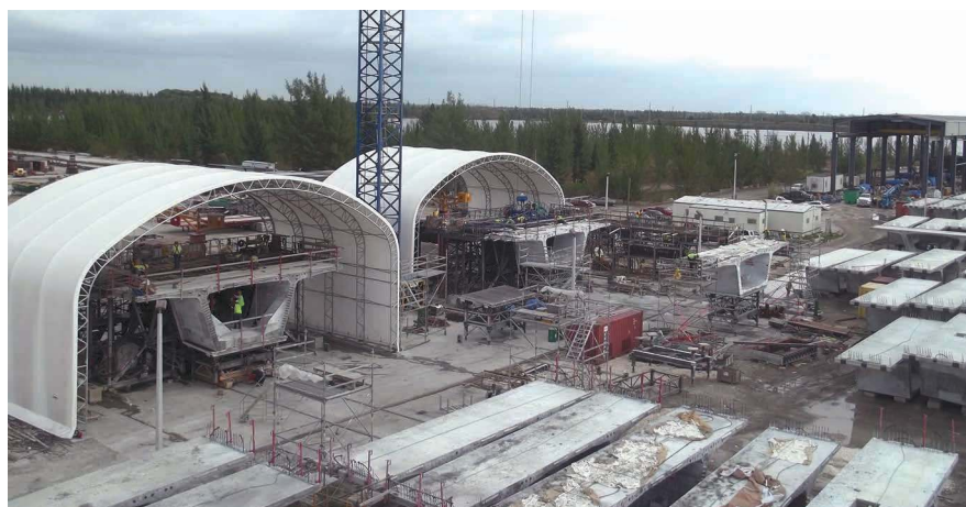
The segment casting yard was located approximately 16 miles away and had two casting cells, which enabled the fabrication of an average of eight segments a week for a total of 783 segments. Photo: Rizzani De Eccher.
