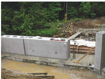
Above: Precast concrete footing installation for the State Route 112 Bridge over Kearney Brook. Right: Precast concrete abutment stem installation. Photos: William E. Dailey Precast LLC.
