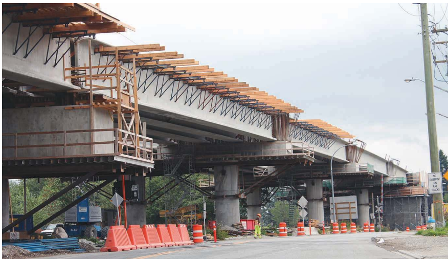
The South Fraser Road project, a public-private partnership completed on a design-build basis, involved 16 bridges along a 25-mile-long, four-lane highway in Vancouver, BC, Canada. The bridges feature mostly precast, prestressed, concrete girders due to site conditions and the ability to reduce costs by repeating the design and gaining efficiencies of scale. From top, Ladner Trunk Road, Highway 99, and BNSF viaduct.
