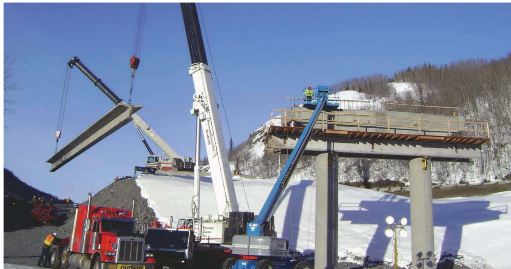
Picking a bulb-tee girder for winter construction of the Hicks Creek Bridge.
