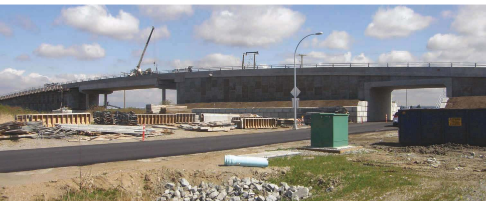
The $12 million 80 th Street Overpass in Delta, BC, Canada, is a design-build project encompassing 500 ft of road upgrades, retaining wall designs using lightweight backfills, and a 107-ft-long concrete bridge.
