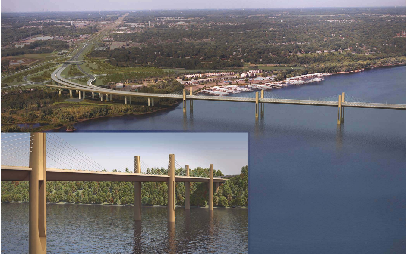
The St. Croix River Crossing from Oak Park Heights, Minn., to St. Joseph, Wis., features an extradosed bridge design, in which post-tensioned box-girders are supplemented with post-tensioning outside the box sections. The external post-tensioning helps support the loads but provides a shallower cable inclination and shorter towers.
