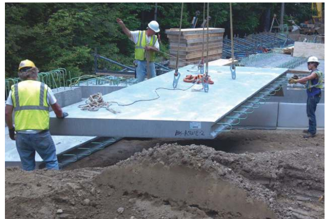
Precast concrete approach slab installation for the State Route 112 Bridge over Kearney Brook. Photo: William E. Dailey Precast LLC.
