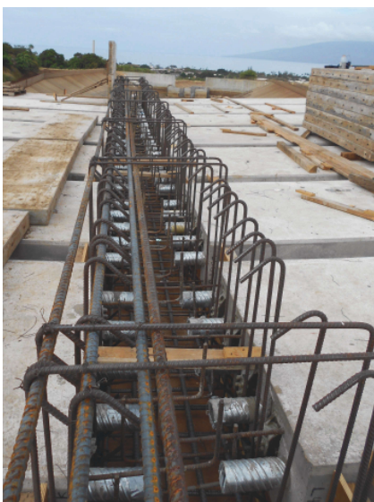
Continuous post-tensioning ducts are spliced at the stiffener beam of the bottom chord. Photo: Eric Matsumoto.
