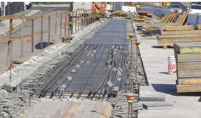
Tee-beam strengthening.
