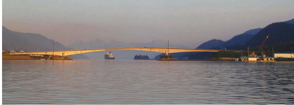
The Gastineau Channel Bridge, as seen from a kayak at sunset.
