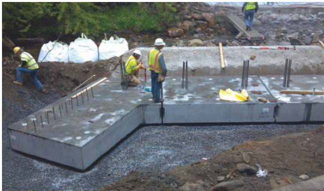
Above: Precast concrete footing installation for the State Route 112 Bridge over Kearney Brook. Right: Precast concrete abutment stem installation. Photos: William E. Dailey Precast LLC.
