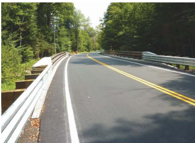
State Route 112 Bridge over Kearney Brook. Photo: Massachusetts Department of Transportation.
