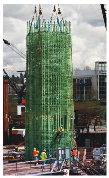
ASTM A775 reinforcing steel being placed for the Willamette River Bridge in Portland, Ore. Photo: Harris Rebar, Auburn.
