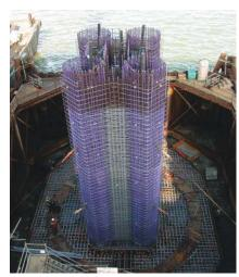
ASTM A936 reinforcing steel used in the San Francisco - Oakland Bay Bridge. Photo: Caltrans.
