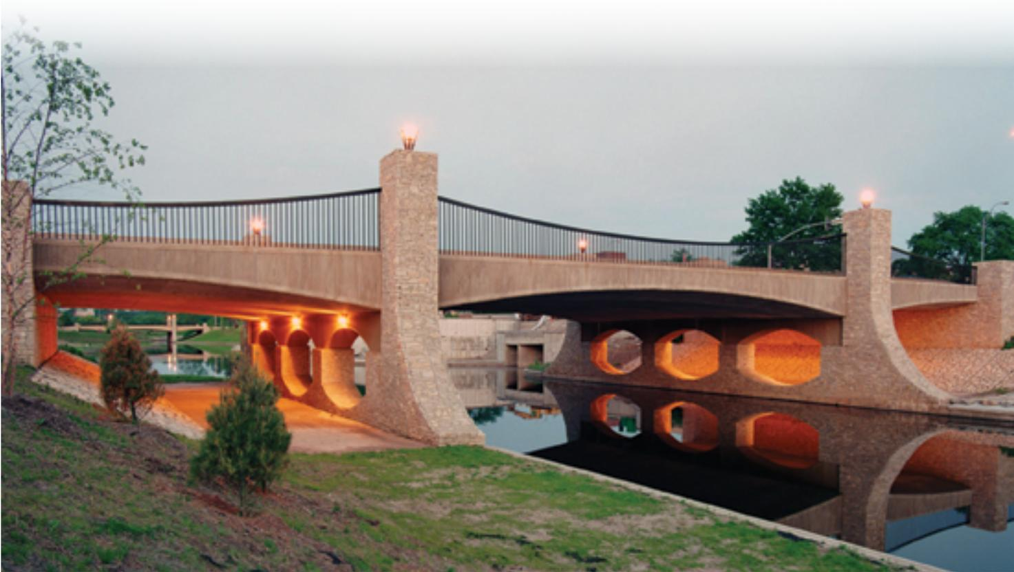
Rockhill Road over Brush Creek, in Kansas City, Mo., was constructed with cast-in-place concrete box beams.
