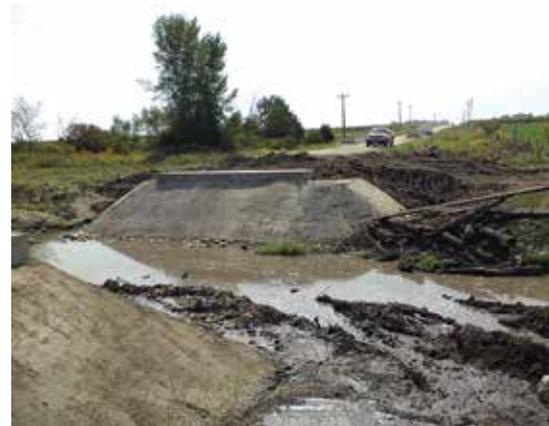
Compacted concrete on geosynthetic reinforced soil abutments on Jakway Park Bridge. Photo: Buchanan County.
