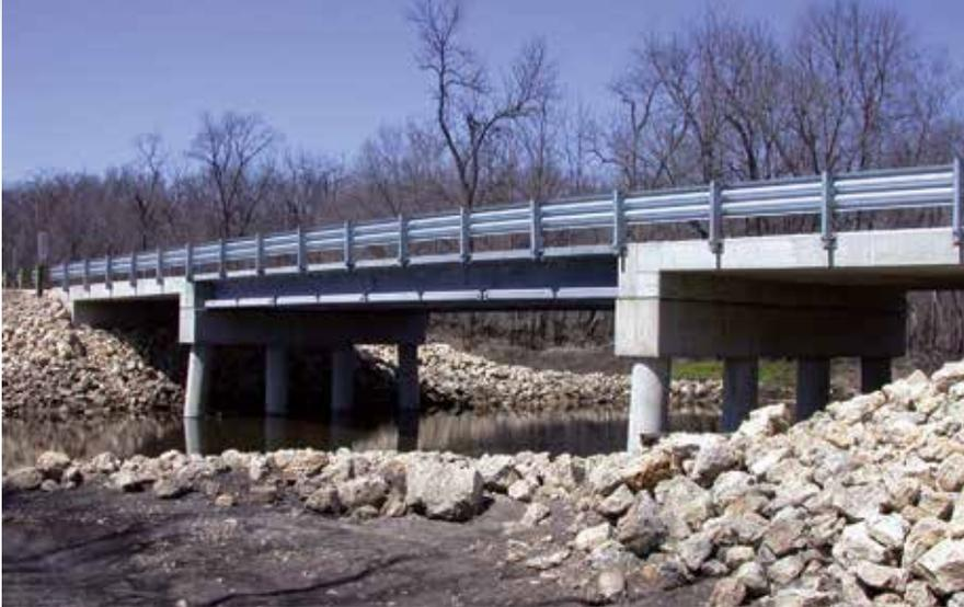
Ultra-high-performance concrete was used in the Pi-shaped girders of the center span of the Jakway Park Bridge. Photo: Iowa Department of Transportation.
