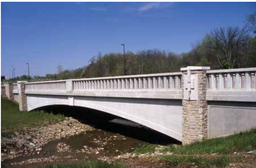
The Emerald Parkway over North Fork Indian Run in Dublin, Ohio, consists of twin, 95-ft-long single-span, concrete box-beam bridges. Detailing included decorative precast concrete arch fascia panels, ashlar limestone facing on abutments, and aesthetic concrete railings. Photo: Burgess & Niple.
