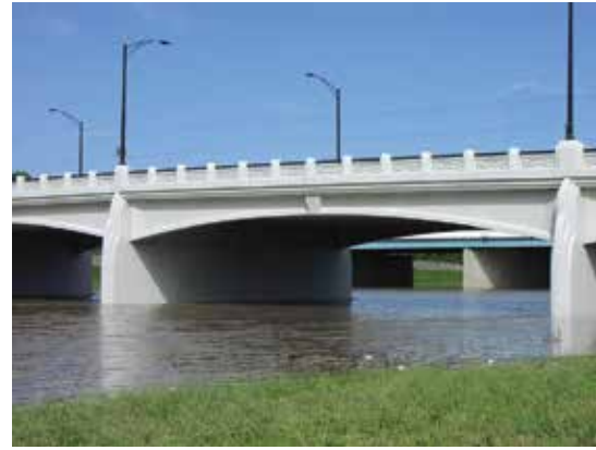
The Fifth Street Bridge in Dayton, Ohio, used haunched exterior girders to invoke the appearance of the original closed spandrel arch bridge. Photo: Henry G. Russell Inc.
