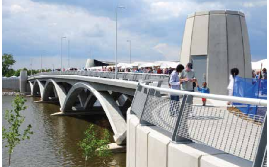
The 568-ft-long Rich Street Bridge in Columbus, Ohio, features precast, post-tensioned lightweight concrete rib arches, with reinforced concrete piers and abutments. Photo: Burgess & Niple.
