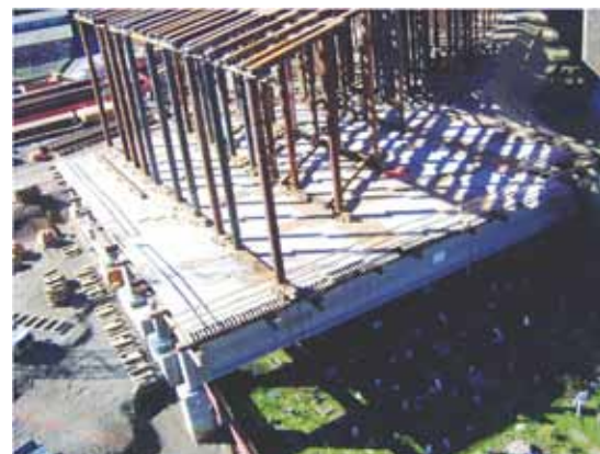
Placing concrete in the soffit of the box girder.
