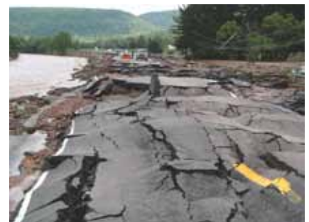
Significant flood damage sustained in north central Pennsylvania with the combined rains of Hurricane Irene and Tropical Storm Lee during fall of 2011. Photos: PennDOT District 3 engineering staff.
