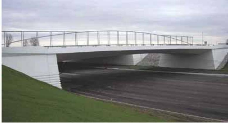
RW Armstrong's transportation team often works closely with its aviation team, such as at the Port Columbus International Airport in Columbus, Ohio, where cast-in-place, post-tensioned, variable-depth box girders were used to create a new taxiway. The project was built on grade, then soil excavated from beneath it to avoid needing falsework.
