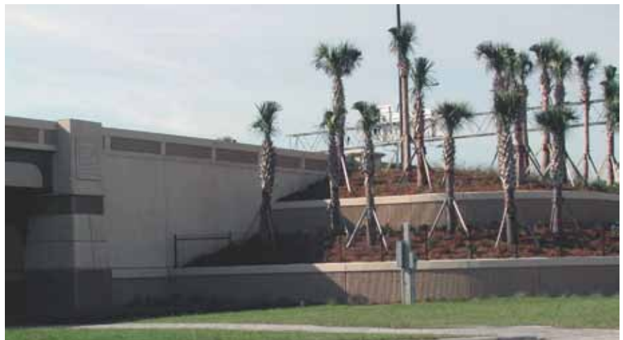
Decorative architectural precast concrete panels were used on the expressway widening through downtown Orlando.
