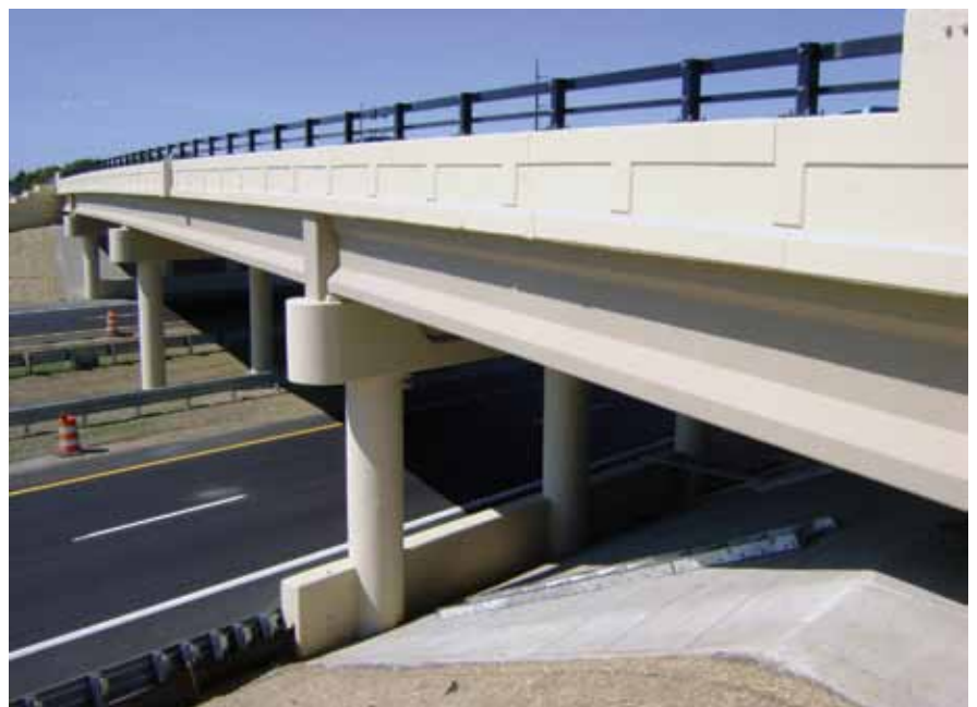
The Parkview Avenue Bridge was designed as a total precast concrete structure to explore the concepts of accelerated bridge construction.
