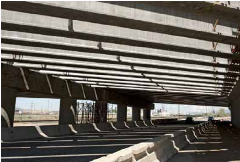
All girders in place on both bridges. Photo: Hanson Structural Precast.
