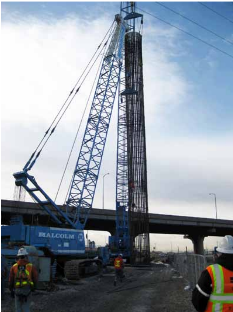
Placing reinforcing cage for 9-ft 2-in.-diameter, 120-ft-long drilled shaft. Photo: Kiewit/Clyde.
