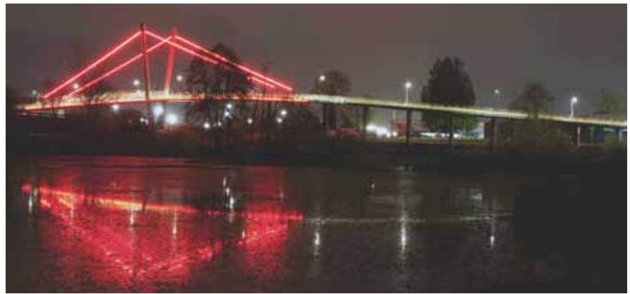
The Delta Ponds Pedestrian Bridge looking over Delta Ponds. Red LED lighting along the deck edge and the top stay create a stunning effect at night.
