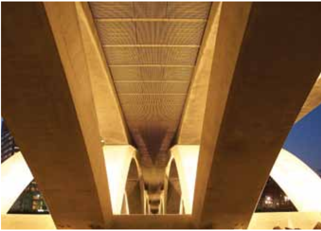
The fiber reinforced grating conceals all the utilities under the deck of the Rich Street Bridge. Photo: Ohio Department of Transportation District 6.
