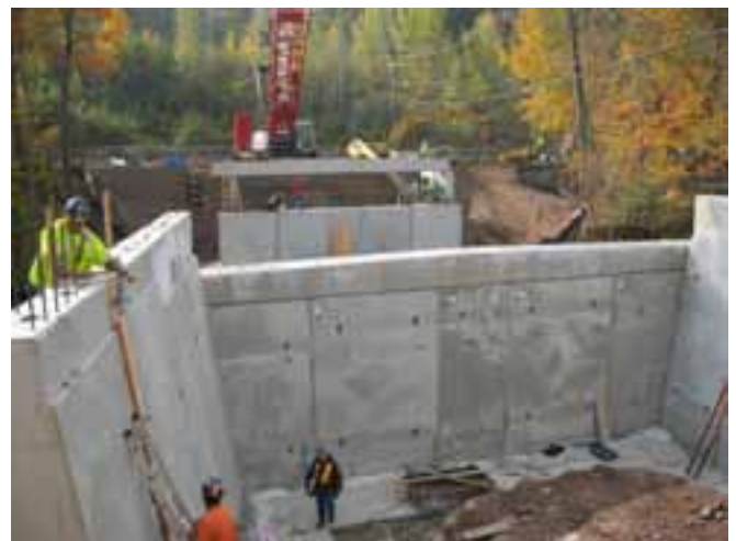
Precast abutment and wingwalls were placed and braced. Vertical form boards were clamped over the joints in two locations to grout the shear keys full. Next, the bridge seat beam will be placed on the abutment walls. Photo: Arborio Corporation.
