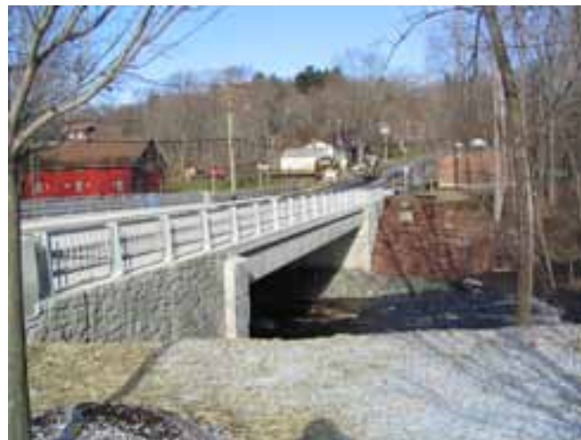
The handsome new South Maple Street Bridge features an ashlar stone texture cast on the wingwalls. Photo: Hoyle, Tanner & Associates Inc.
