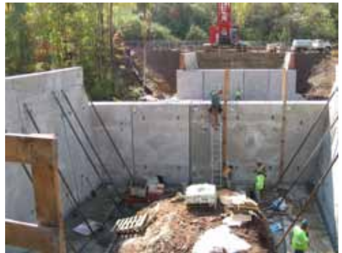
Precast abutment and wingwalls were placed and braced. Vertical form boards were clamped over the joints in two locations to grout the shear keys full. Next, the bridge seat beam will be placed on the abutment walls. Photo: Arborio Corporation.
