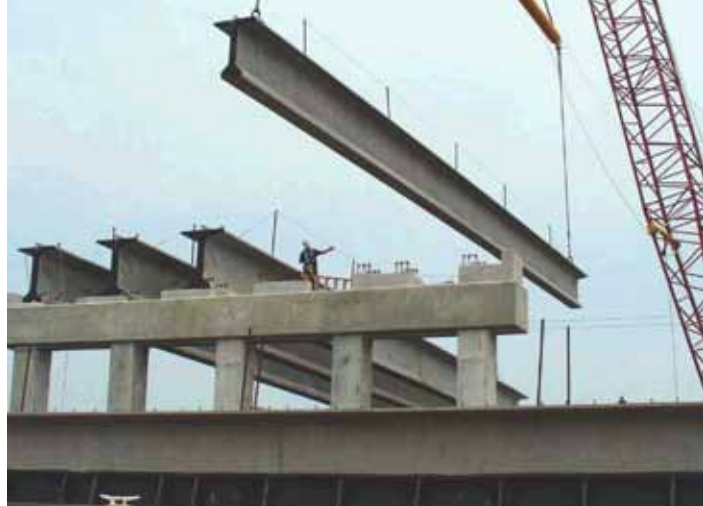
The typical spans included 135-ft-long, 78-in.-deep Florida Bulb-tee beams set on precast pile caps on 36-in.-square, hollow, precast, prestressed concrete piles.
