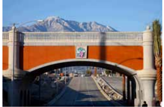
Beautiful Cucamonga Peak rises majestically beyond the completed Haven Avenue Grade Separation Bridge. Photo: PBS&J, an Atkins company.
