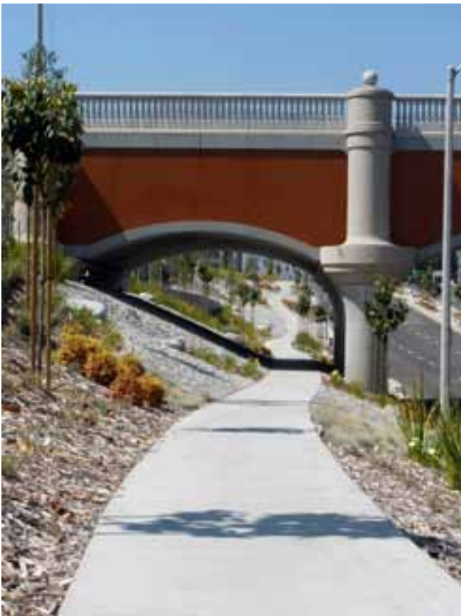
A pedestrian way alongside Haven Avenue passes beneath the new grade separation. Photo: City of Rancho Cucamonga.
